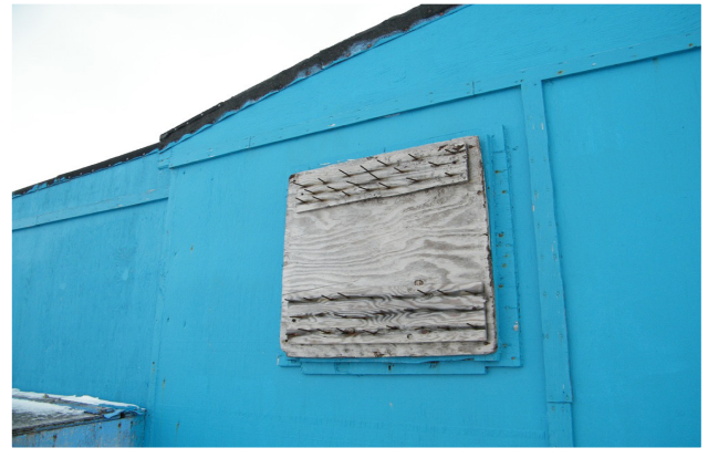
A cabin window covered by a bear board
