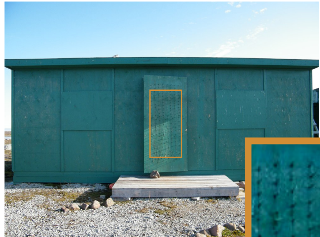
The main cabin door is protected by a bear board on hinges. The bear board door can be removed when the cabin is being used regularly
