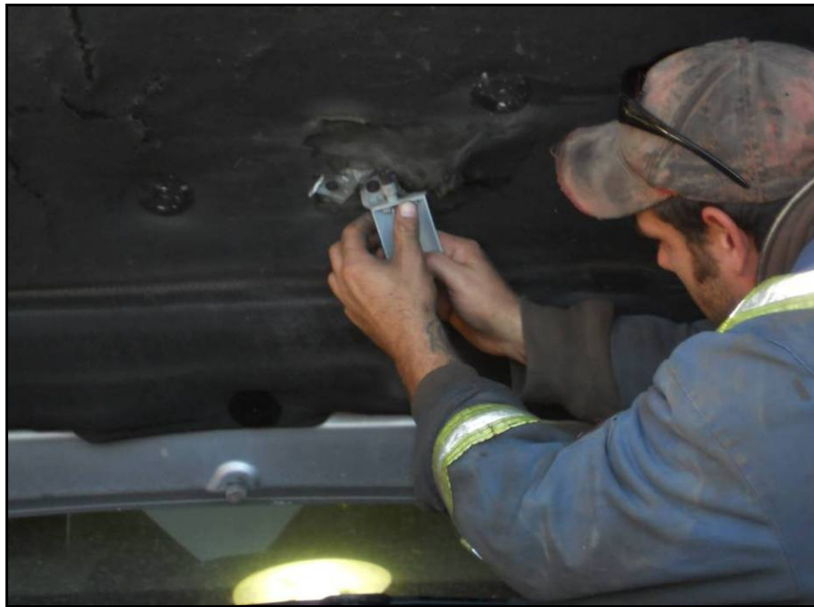
Figure 15: Example of Removing Light Assembly Containing a Mercury Switch
