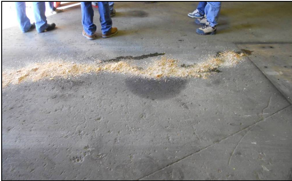
Figure 2: Absorbent Material place over Spilled Vehicle Fluids
