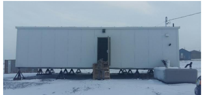
1 Sanikiluaq Community Freezer
